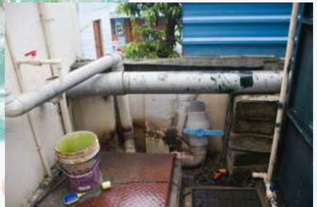
Rainwater Harvesting Sumps
