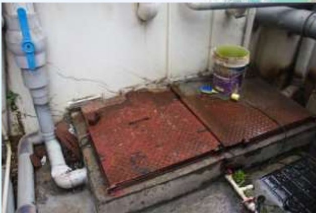
Rainwater Harvesting Sumps
